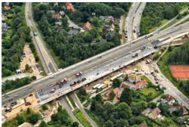
Skovbrynet Highway Bridge Project, Greater Copenhagen
